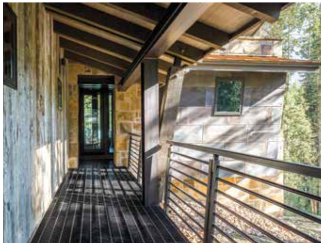
(clockwise from left) The formal entrance to “mountain modern” masterpiece 109 Polecat Lane; steel walkways, beams and railings connect the outdoors and indoors and are a key design feature of the home.
